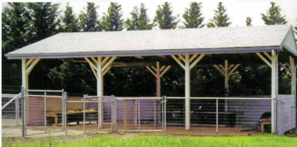
High, open shelters complement the style of the main house, and provide adequate shelter in the mild Southern California climate. Gates inside and outside the shelter provided a variety of options to keep animals together or apart.
